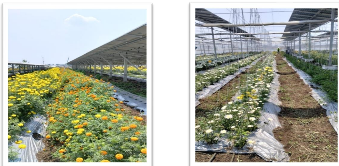
Figure 26: Flower crops under solar panel (Manwath AgriPV plant, Maharashtra)
