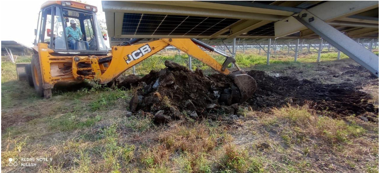
Figure 6 : Excavator removing rocks
