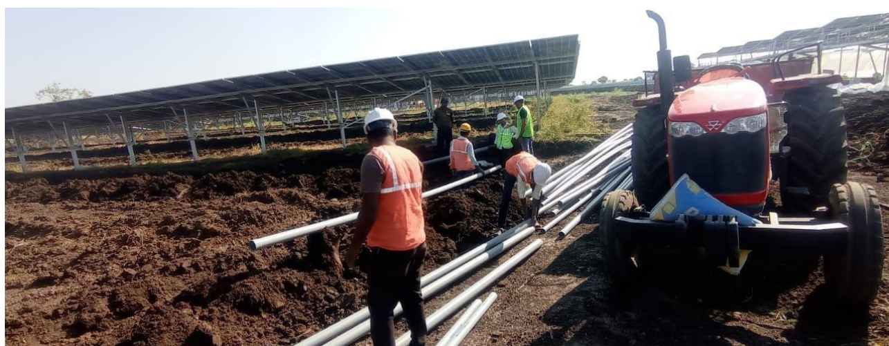
Figure 9: Installation of pipes for borewell
