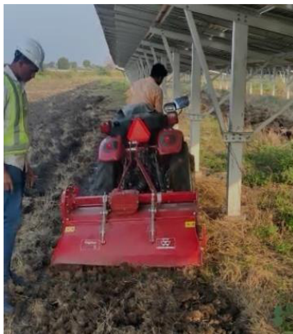
Figure 4 & 5: Concrete removal & site cleaning
