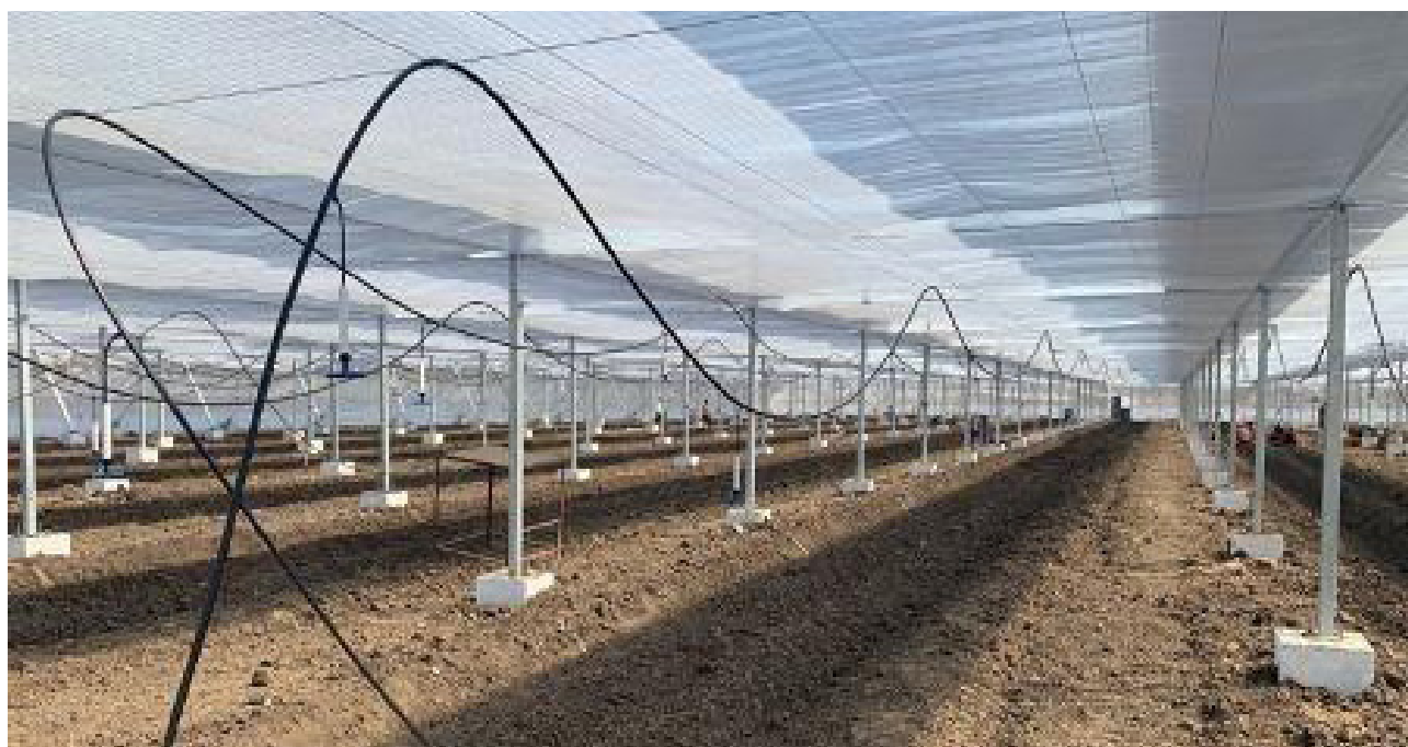
Figure 8: Irrigation & Electricals installation
