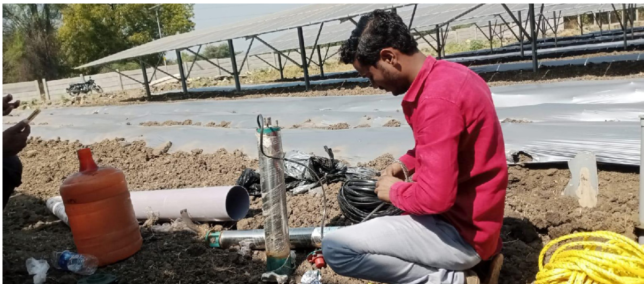
Figure 10: Installation of borewell
