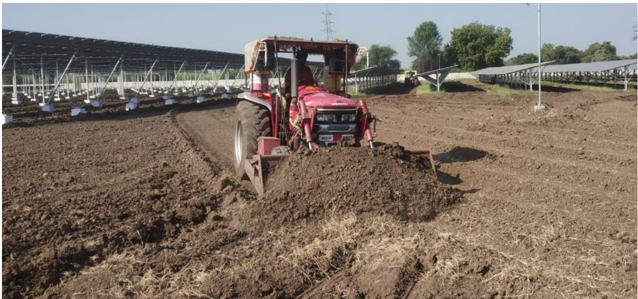
Figure 7 : Levelling of soil
