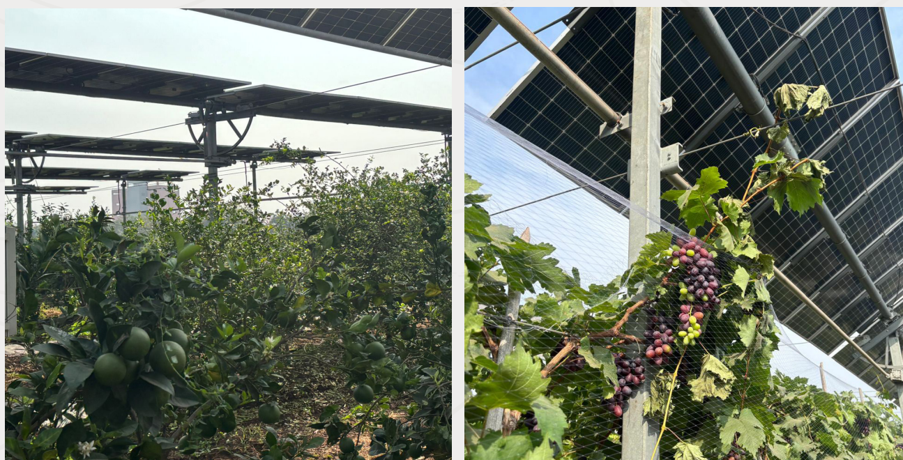
Figure 34. Citrus fruits and Grapes plantation under elevated solar PV (Credit: GIZ, Sahyadri Farms)
