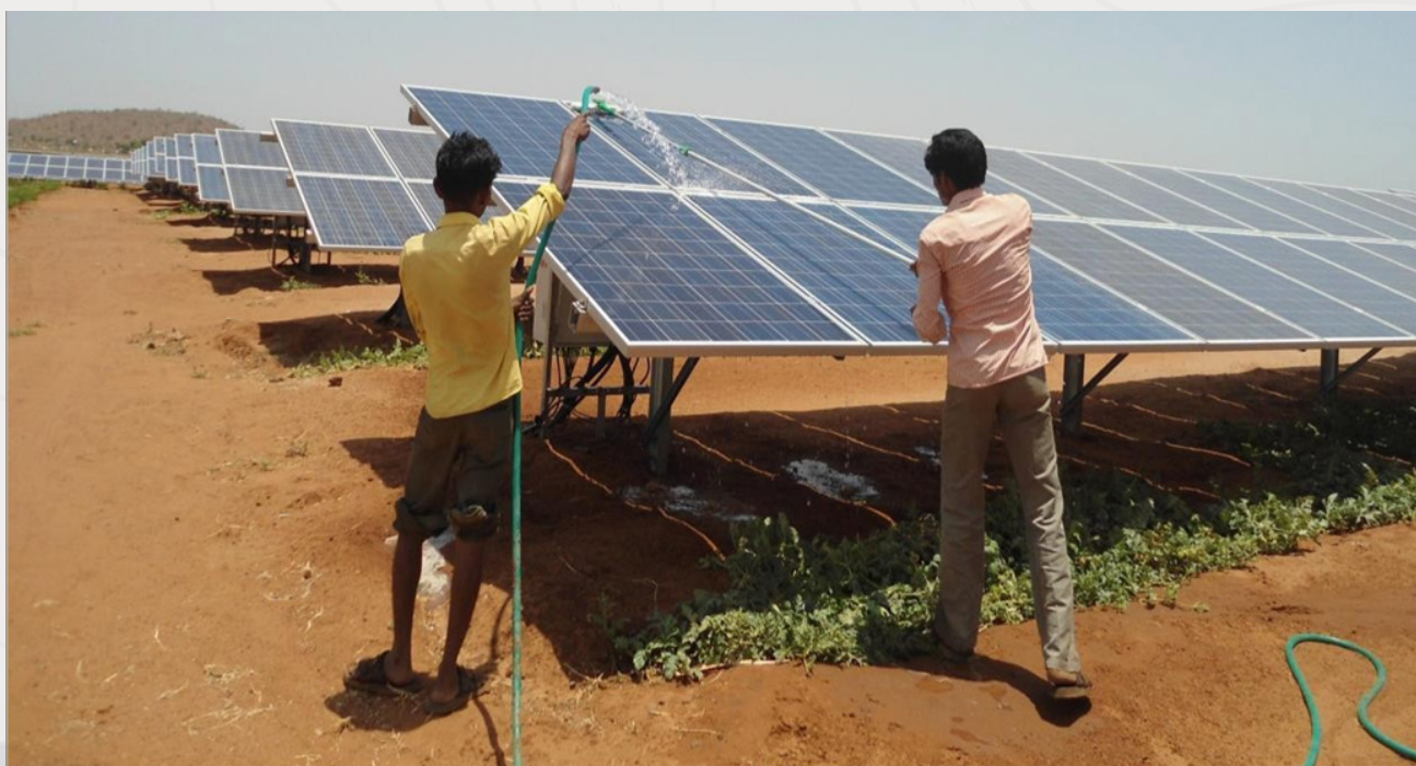
Figure 33. Cleaning of Solar PV'
