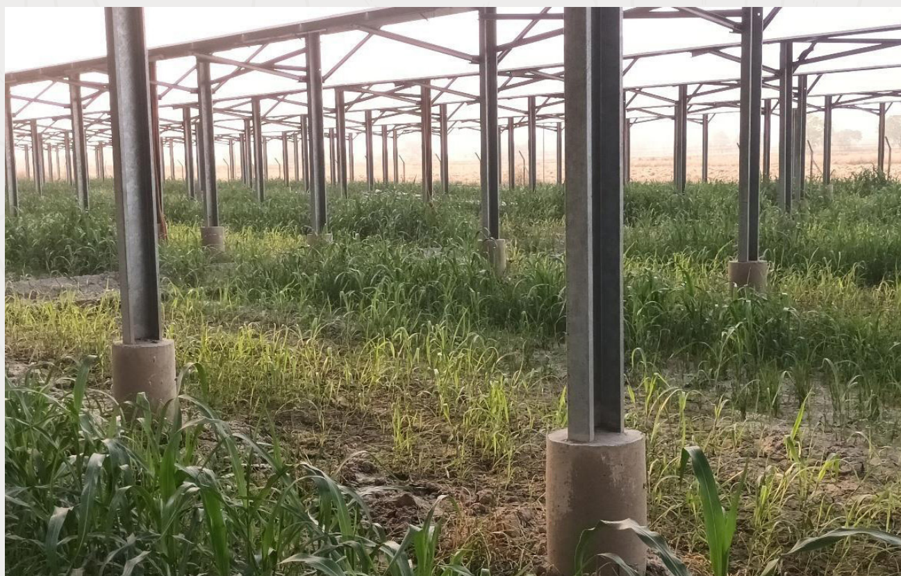
Figure 3. Crops grown at the 4.2 MW plant by Talf Solar
