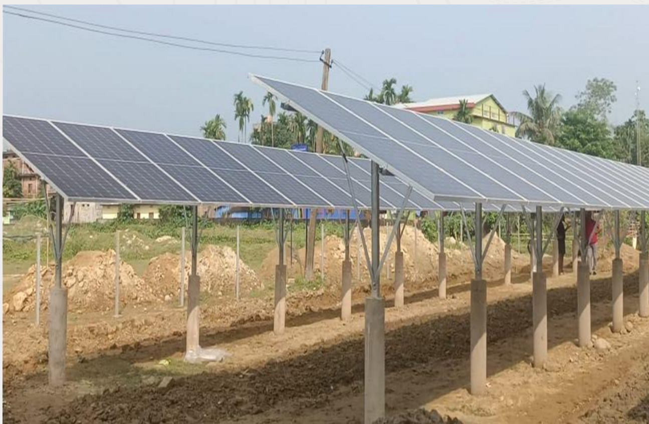
Figure 57. Panel structures of the 50KW- Hailakandi Agrivoltaics project, Assam
