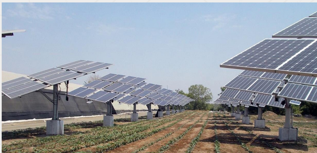
Figure 39. Agrivoltaics with 2-axis tracking and drip irrigation (Credit: Jain Irrigation)
