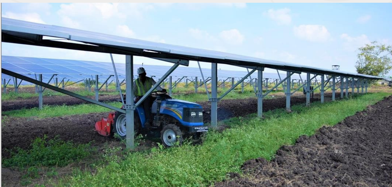
Figure 20. Soil preparation at section III (below and interspace) at Agrivoltaics plant near Parbhani (Credit: GIZ)
