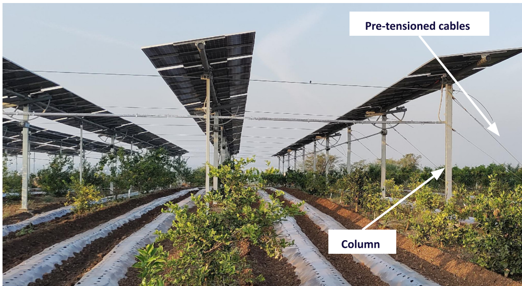
Cable-stabilised array, Sahyadri Farms, Nashik
